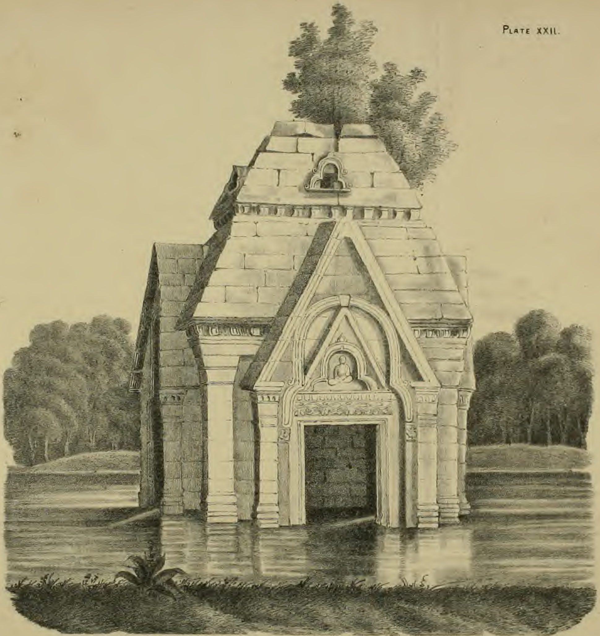
VIEW OF THE TEMPLE OF MERUWARDHANASWAMI AT PANDRETHAN, KASHMIR. A.D. 913-921.
