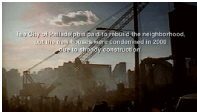
[The City of Philadelphia paid to rebuild the neighborhood, but the new houses were condemned in 2000 due to shoddy construction.]
