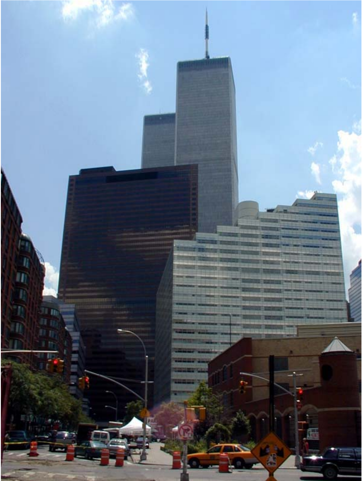
World Trade Center building 7 is the dark building before the looming Twin Towers. The light terraced building in front of it is 101 Barclay Street (view from Greenwich Street).
